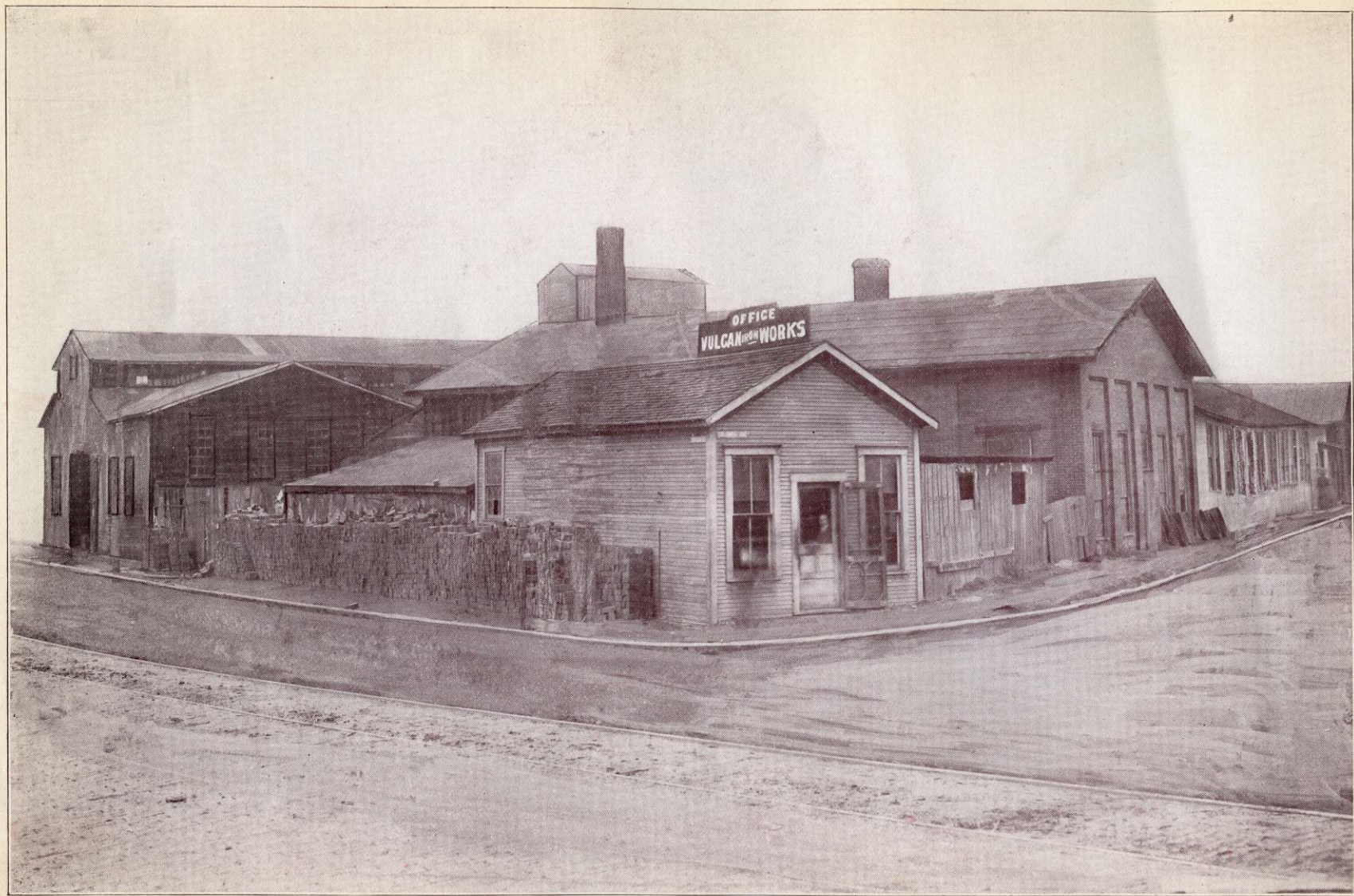
Vulcan Iron Works Boiler Works, Machine Shops and Foundry.
