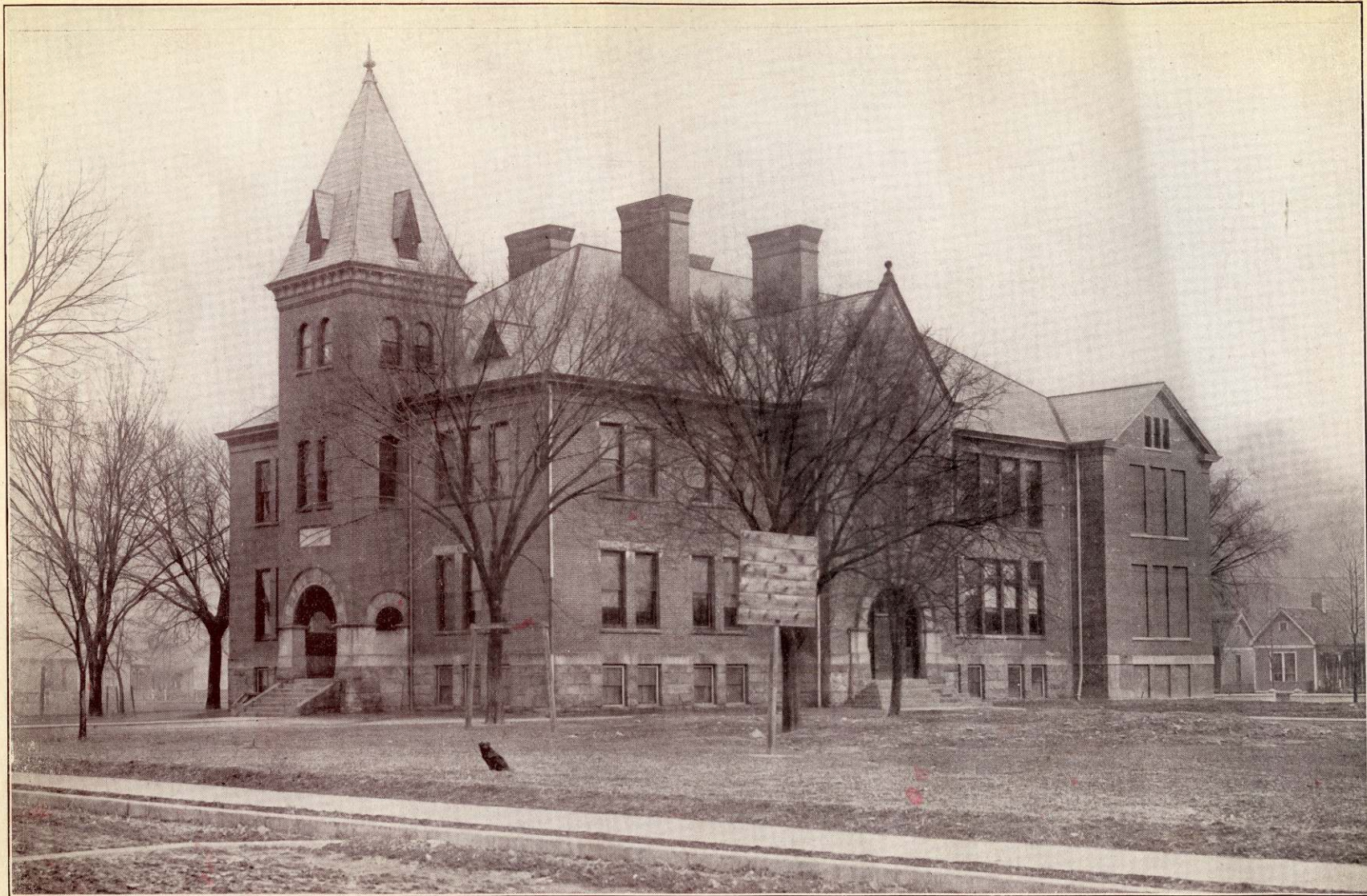
Lincoln School Building
