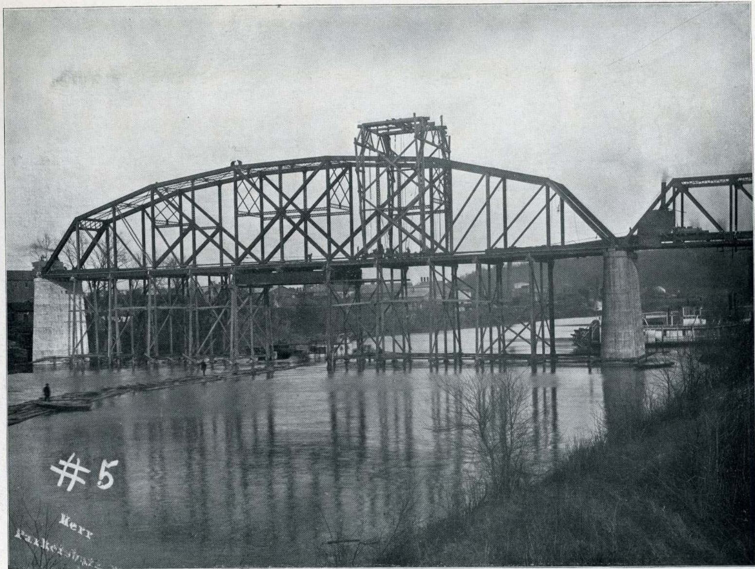
New East Street Bridge, Crossing Little Kanawha River.
