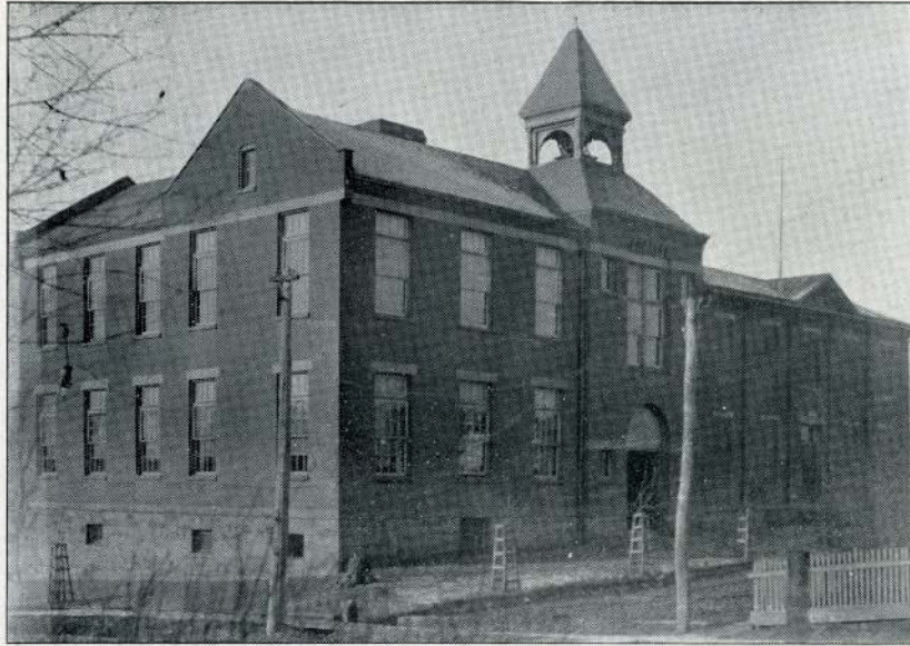
The Jefferson School, Parkersburg,
